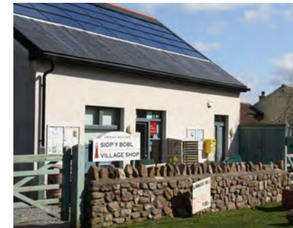
Left: PV installation Llanmadoc
