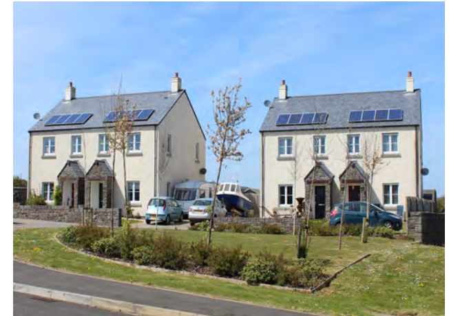
Above: Affordable Housing, Scurlage
