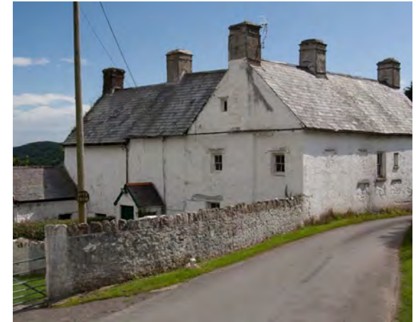
Above: Pitt Farm, above Oxwich is an example of a former small manor house. Sharing a number of characteristics of traditional farm houses such as small windows, rendered walls and slated roof
