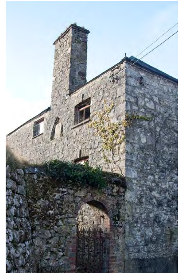
Above: Lower Mill, Llanrhidian: Grade II
