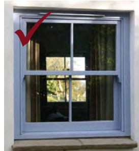
Left: timber sash style painted window
