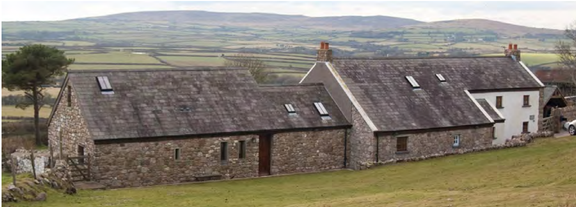
Above: conversion which has respected the character of the existing building, in terms of openings and roof detailing, Reynoldston
