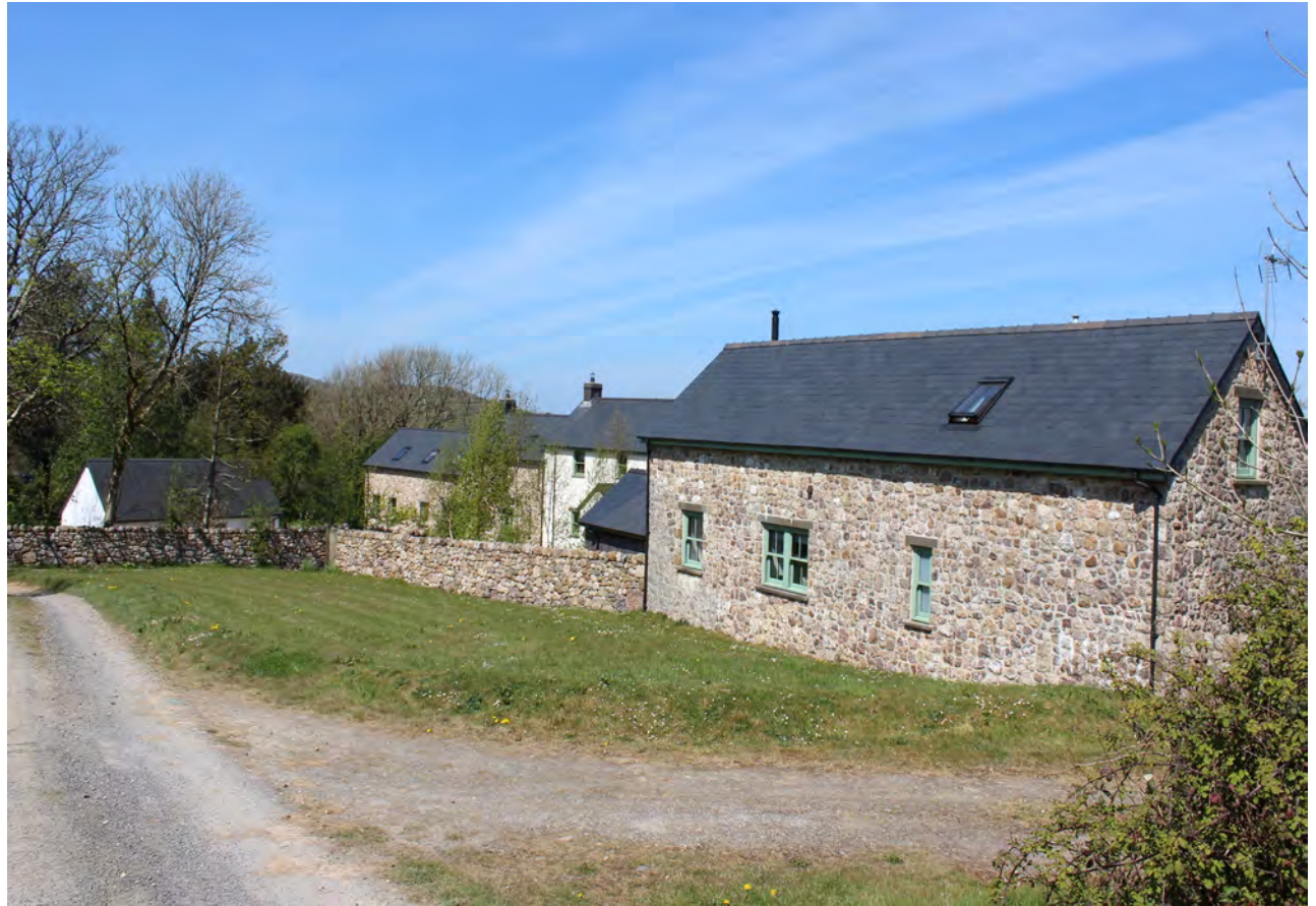
Above: Replacement farmhouse and conversion of outbuildings to provide dwelling house and holiday accommodation, Hill End Farm, Reynoldston. The stone wall, grass verge and planting enhance the development.
