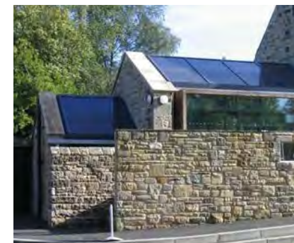
Left: PV installation integral to building design
