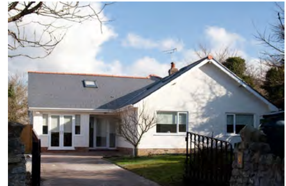
Above: recently renovated adjacent property
