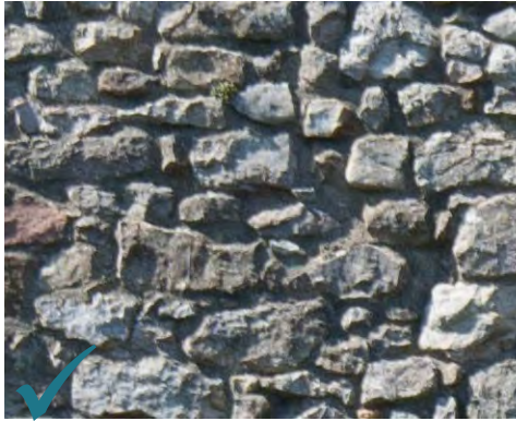
Traditional pointing to stone wall
