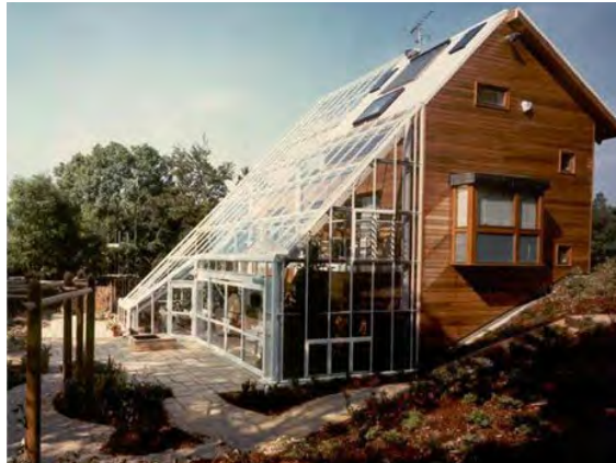
Above: BRE Integer House, Garston, Watford
