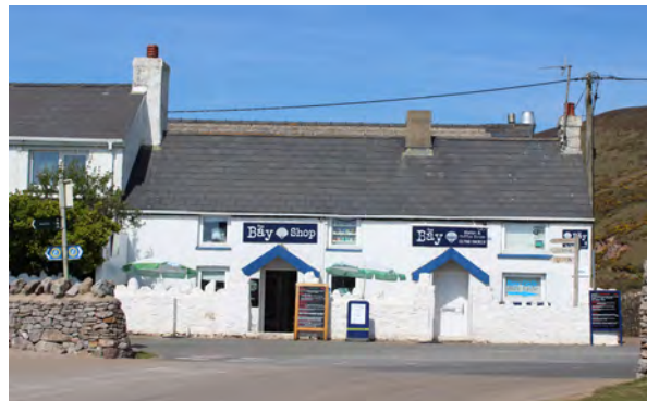
Below: Image shows a variety of signage - highway, Rights of Way, advertising and commercial
