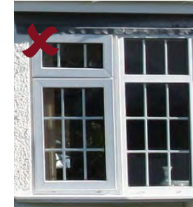
Left: uPVC opening and fixed casement window with overly wide frames
