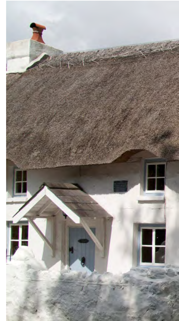
Above: The Nook, Oxwich: Grade II
