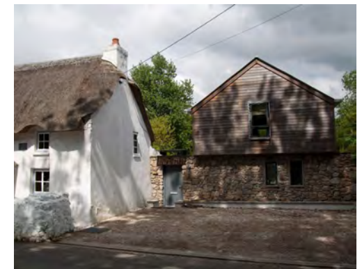
Above: contemporary extension to a Grade II listed thatched cottage, Oxwich
