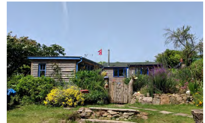
Below: Chalet at Holts Field
