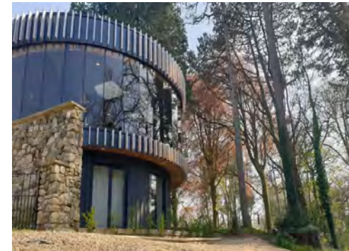
Right: Contemporary extension at Fairyhil @Raum Architects
