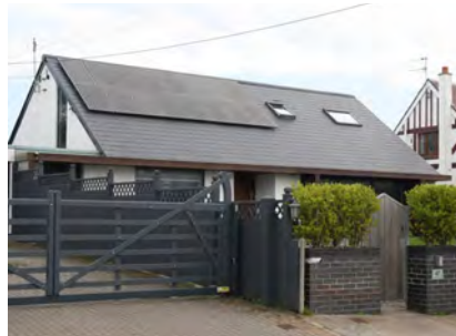
Above: Photovoltaics to roof, Southgate
