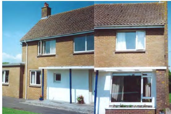
Above: before renovation
