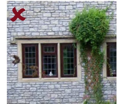
Above: 20th century development which has poorly chosen stone, in terms of both colour and size, and inappropriate mortar colour and pointing style
