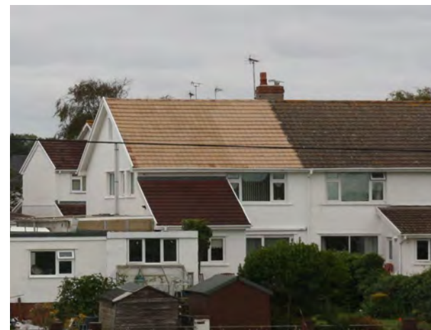
Above and below: Extensions and re-roofing can result in the introduction of numerous, inappropriate or unsympathetic materials or colours, which can have a negative impact upon an individual building, character of an area, or key views.
