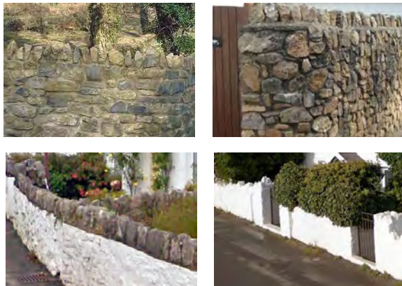
Top: appropriate types of stone walling Bottom: different styles of whitewash finish
