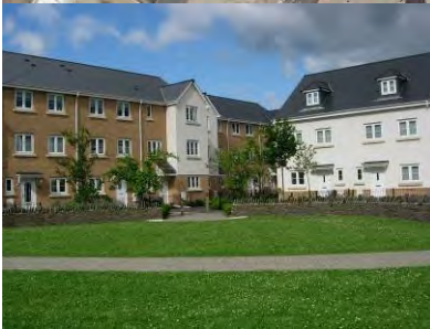
Bryngwyn Village, Gorseinon. Typically 40 dwellings per hectare. Mixture of houses with gardens and flats, including open spaces*
