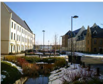
Example of SuDs integrated as a focal point in the public realm (Upton, Northampton)
