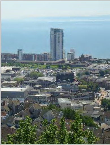
Meridian Tower—creates an landmark building in the Maritime Quarter which maximises density in the city centre.
