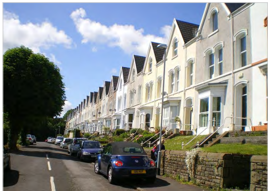
Local examples of building detailing in Swansea— gables & bay windows
