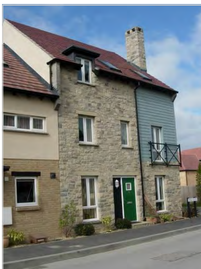
Example of contrast in the streetscene achieved through a change in scale and materials.
