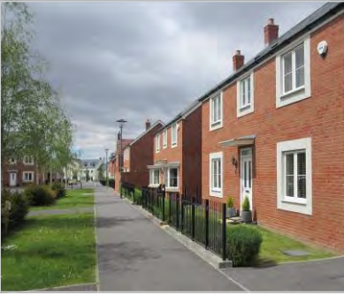
Front gardens and boundaries provide a buffer between the home and the street
