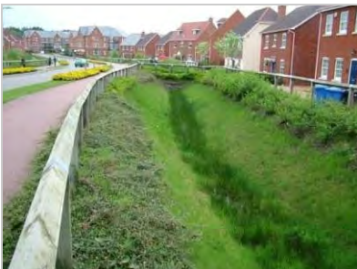
SuDS features can add visual interest and character to schemes in addition to reducing the impact of surface water run-off
