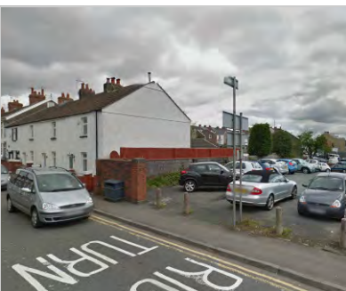
Blank Side elevations onto the public realm do not provide opportunities for natural surveillance
