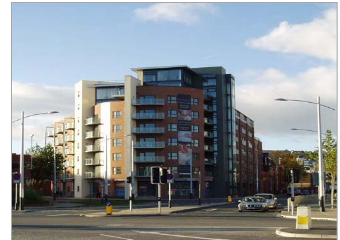
Excelsior Building, Princess Way (9 storeys)
