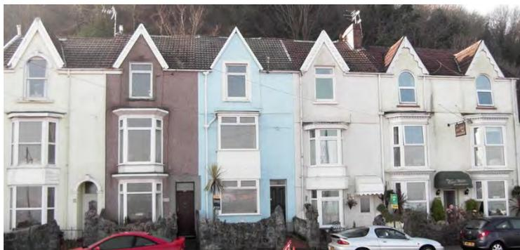
Fig 7.1 This attractive sea front terrace of Victorian houses displays the concerns of gradual change: loss of chimney stacks/pots; replaced gable barge boards; removal of the arched top floor window openings; two inaccurately rebuilt two storey bays; changed window fenestration; door openings and doors have been replaced; and the pebble-dash wall finish does not respect the traditional design.
