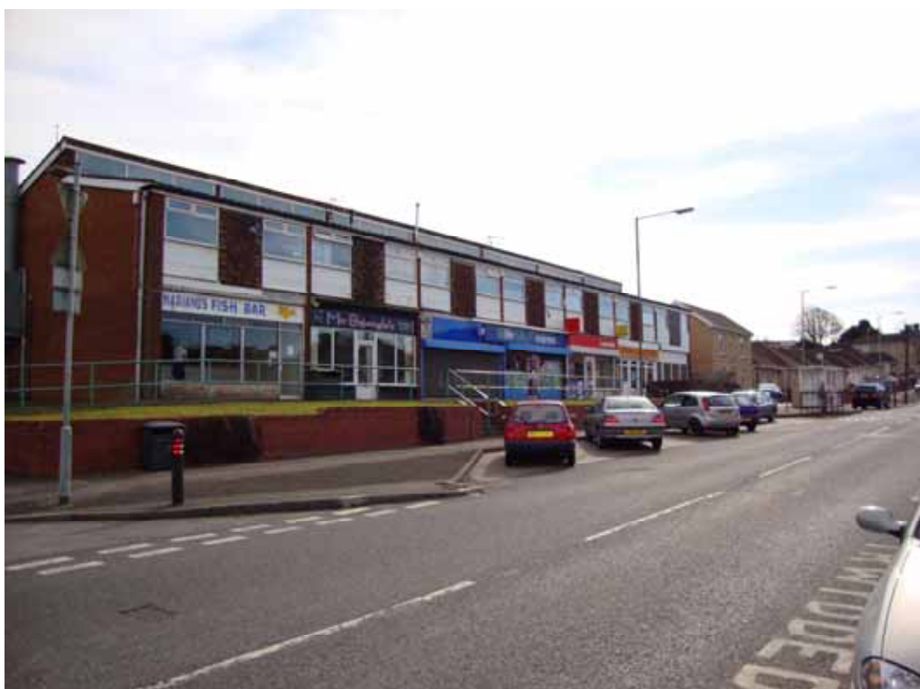
Local Centre at Trallwn Road, Trallwn
