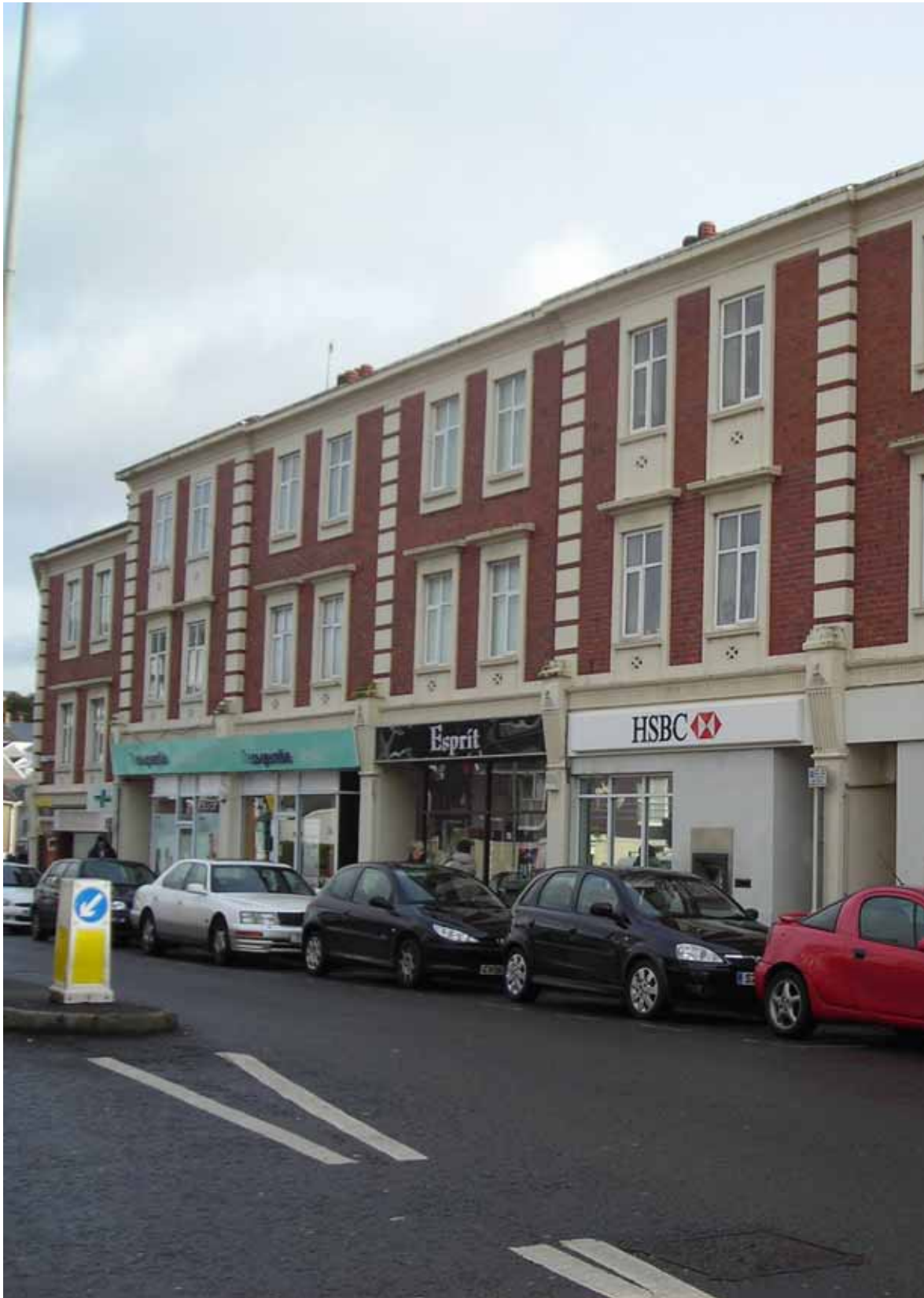
Commercial frontage at Sketty District Centre
