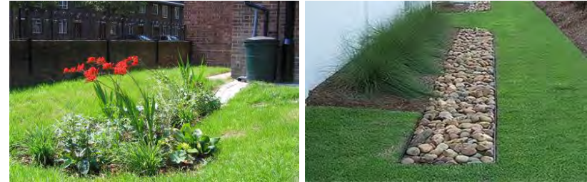
Fig 3.3 Plot level features such as a surface level rain garden (left) and infiltration trenches (right) can be incorporated into developments
