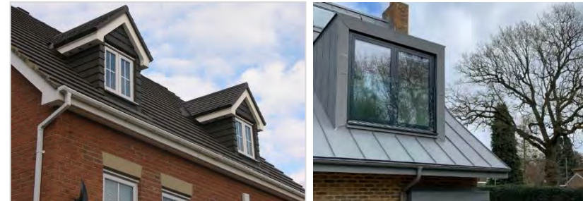
Fig F.7 Small dormers which relate well to the windows below (left) and contemporary dormer of matching roof materials (right)
