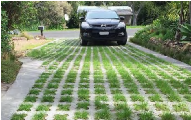
Fig J.1 Permeable block paving driveway with grass
