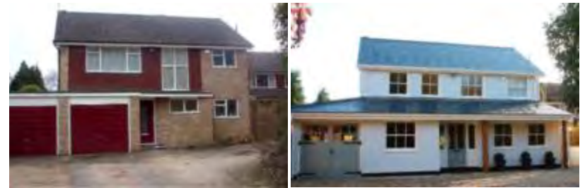
Fig G.2 Enhancement scheme including new roofing materials, windows and render
