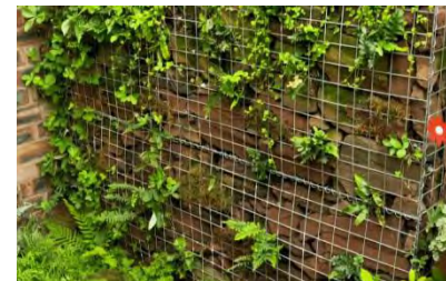
Fig 3.1 Living/Green walls provide multiple benefits including habitats and biodiversity enhancements as well as helping to absorb and hold rainwater to help minimise flooding.
