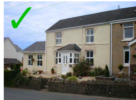
Fig B.4 A single storey extension successfully incorporating the materials, roof pitch and proportion of windows of the original house
