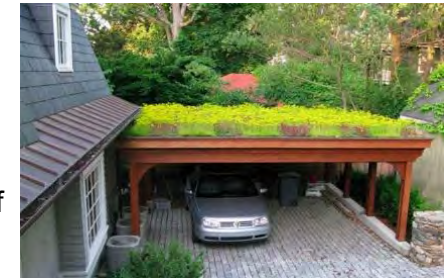
Fig 3.2 Green roofs can be applied to a number of flat or shallow pitched structures
