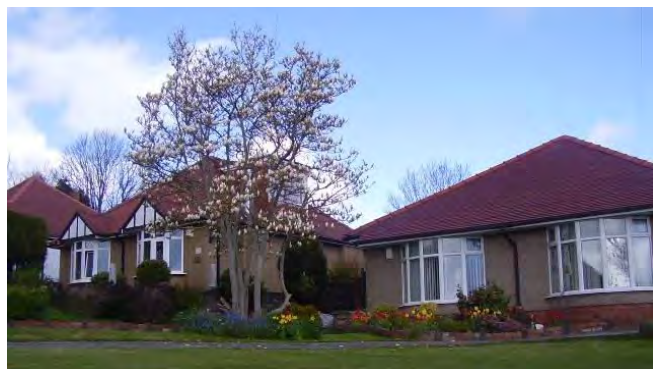
Fig D.1 Bungalows offer accessible accommodation. Any roof alterations must be carefully considered
