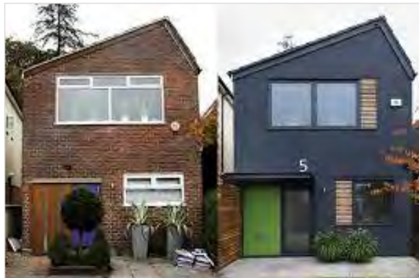
Fig G.5 Enhancement scheme with new openings, contemporary canopy and brick painting
