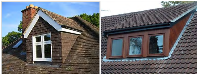
Fig F.3 Gable dormer window (left) and Catslide dormer extension (right)
