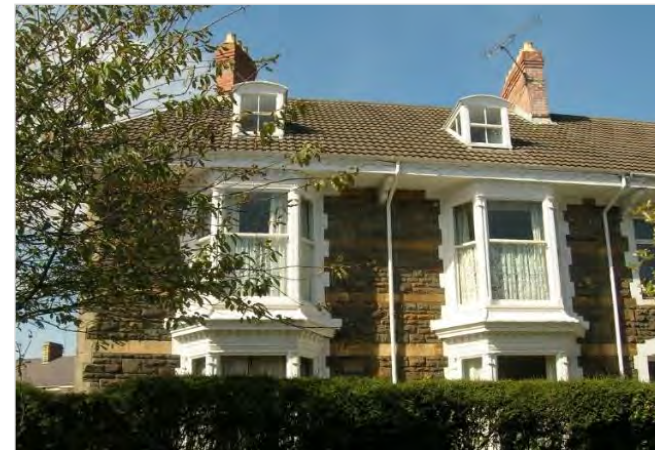
Fig F.2 Original dormer windows respond to the symmetrical character and pattern of openings without dominating the roofplane
