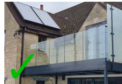
Fig H.3 Contemporary rear balcony extension incorporating privacy screen to protect neighbouring amenity
