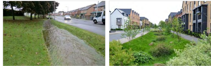
Simple grassed swales convey water during wet weather (left) and a vegetated street swales (right) can improve biodiversity and street character
