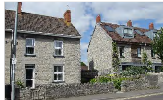
Fig 4.4 Example of infill development that provides a subtle updating of the local vernacular whilst following the established building line and scale.
