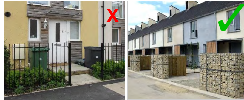
Fig 4.12 Refuse and recycling storage should be well integrated and should not detract from frontages and the public realm.
