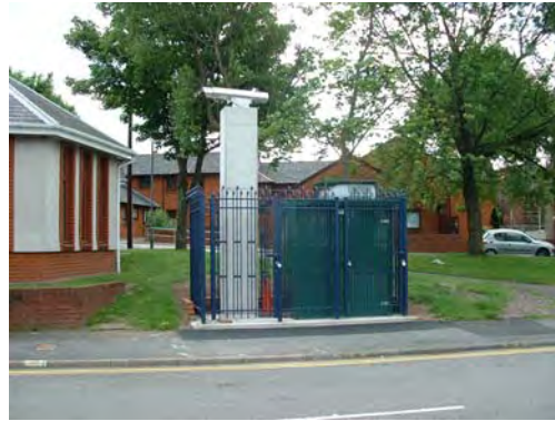
Photo 2 - St Thomas DOAS Receiver Station
