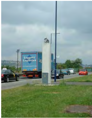
Photo 1 - St Thomas DOAS Transmitter
