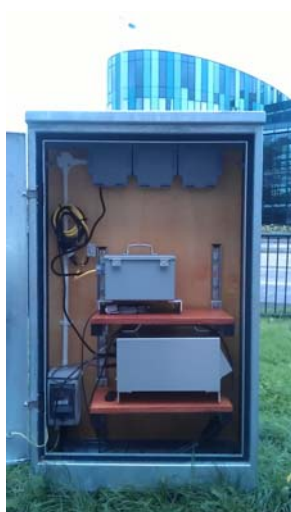
Photo 14- Typical PM 10 Pump Pack
