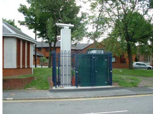
Photo 2 - St Thomas DOAS Receiver Station
