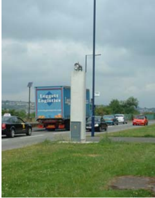
Photo 1 - St Thomas DOAS Transmitter
