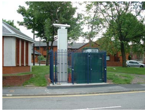
Photo 2 - St Thomas DOAS Receiver Station
