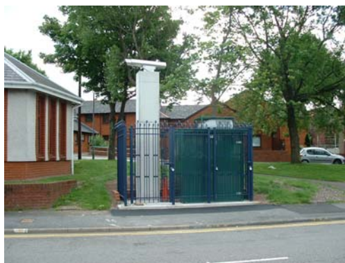
Photo 2 - St Thomas DOAS Receiver Station
