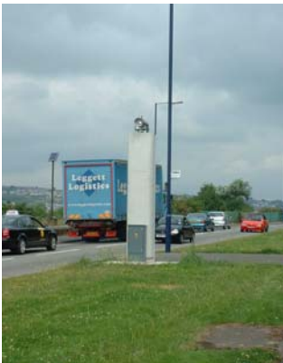
Photo 1 - St Thomas DOAS Transmitter
