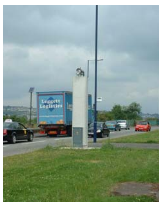
Photo 1 - St Thomas DOAS Transmitter
