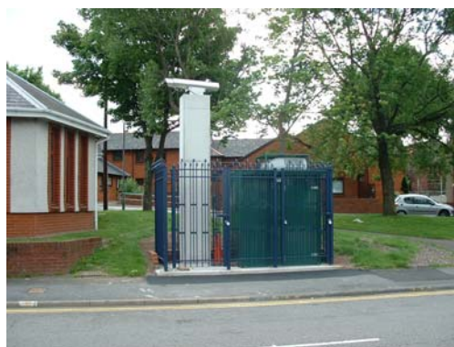
Photo 2 - St Thomas DOAS Receiver Station
