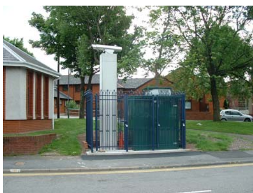
Photo 2 - St Thomas DOAS Receiver Station
