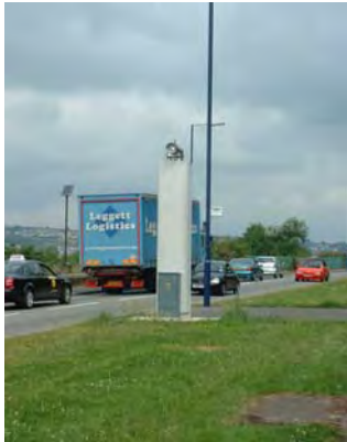
Photo 1 - St Thomas DOAS Transmitter
