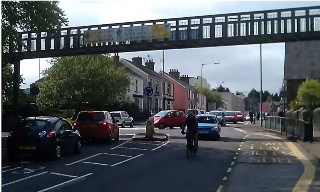
Photo 7 – View looking north to site 7
