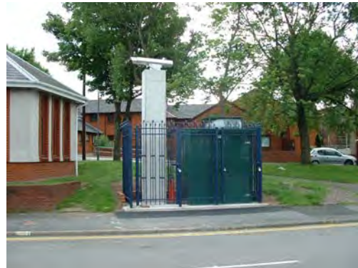
Photo 2 - St Thomas DOAS Receiver Station
