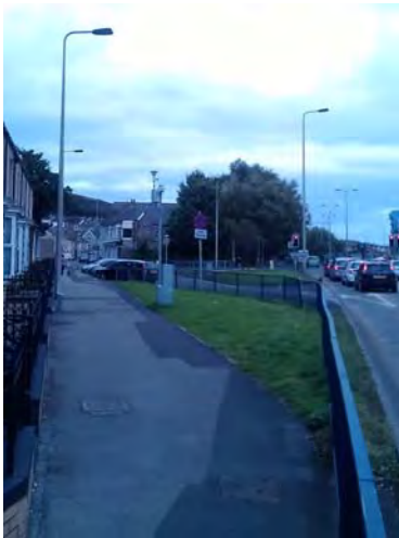
Photo 16 - SA1 PM 10 EBam Installation
