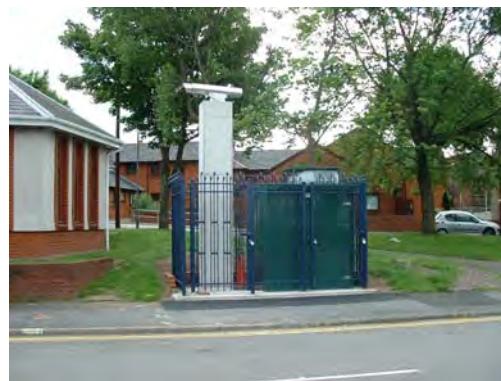
Photo 9 - St Thomas DOAS Receiver Station
