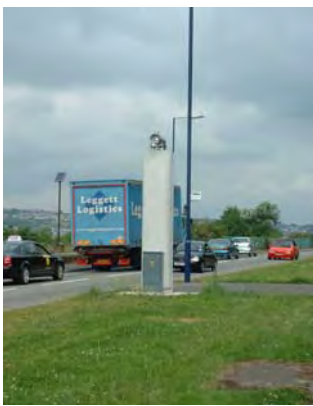
Photo 8 - St Thomas DOAS Transmitter
