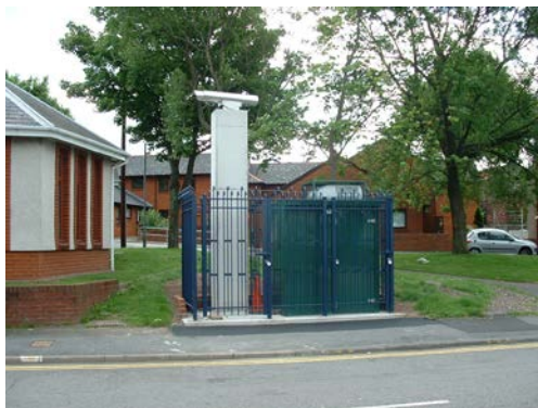
Photo 2 - St Thomas DOAS Receiver Station
