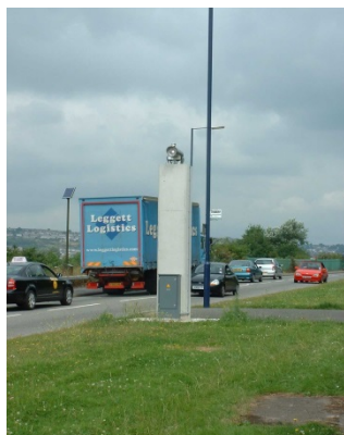
Photo 1 - St Thomas DOAS Transmitter
