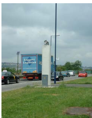
Photo 8 - St Thomas DOAS Transmitter
