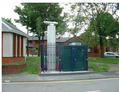
Photo 9 - St Thomas DOAS Receiver Station
