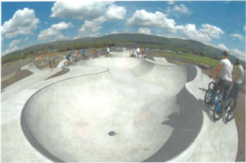
view above road level
