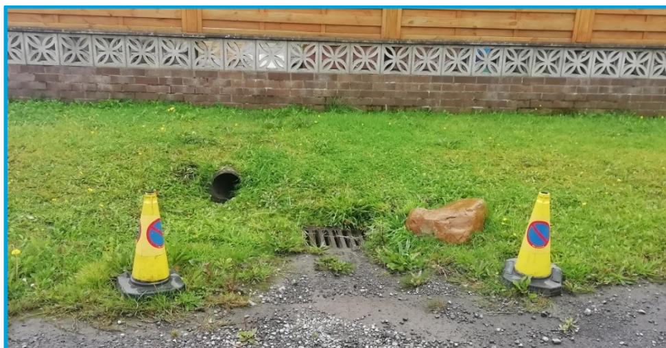
Figure 4-2 – Photograph of gulley and inlet outside No.19 Beryl Road.
