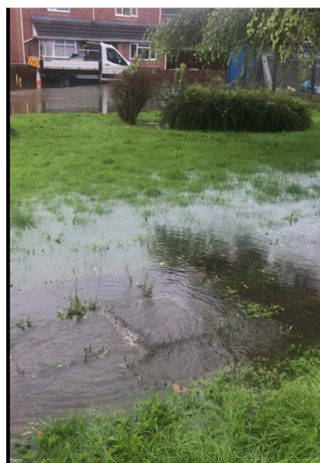
Figure 5-5 – Water 'bubbling-up' from surface water cover at 06:45hrs (video still).
