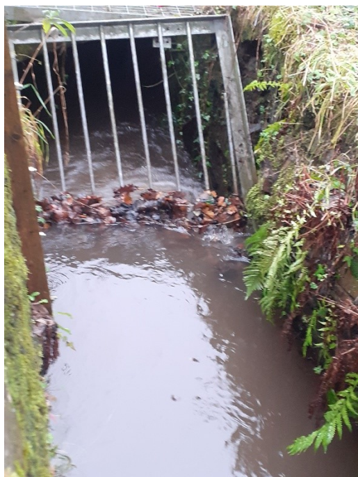
Figure 6-7 – B4603 Pontardawe Road Screen illustrating reduction in water levels following screen clearance on 13 th December 2020.
