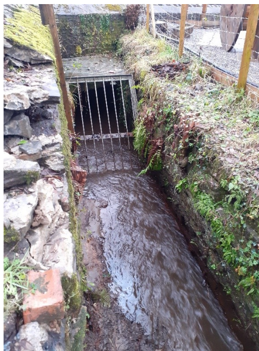
Figure 6-7 – B4603 Pontardawe Road Screen illustrating reduction in water levels following screen clearance on 13 th December 2020.
