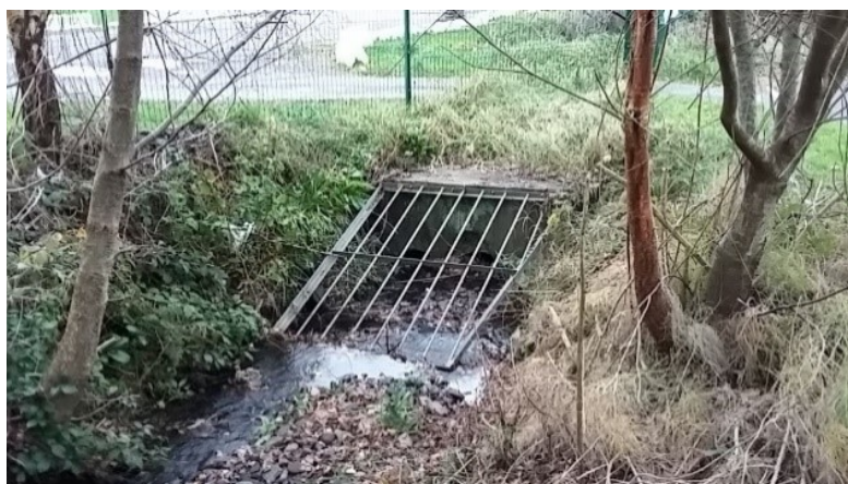
Figure 3-2 – Screen and headwall on short culvert under the Cricket Club access from Park Road/ Waverley Close.
