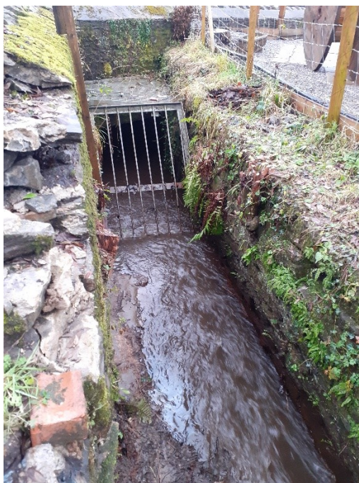
Figure 3-13 – B4603 Pontardawe Road (Men’s Shed) Screen – Culvert entrance to canal through Mond Works.
